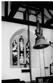
The tolling bell being hoisted back after repair (1999)
